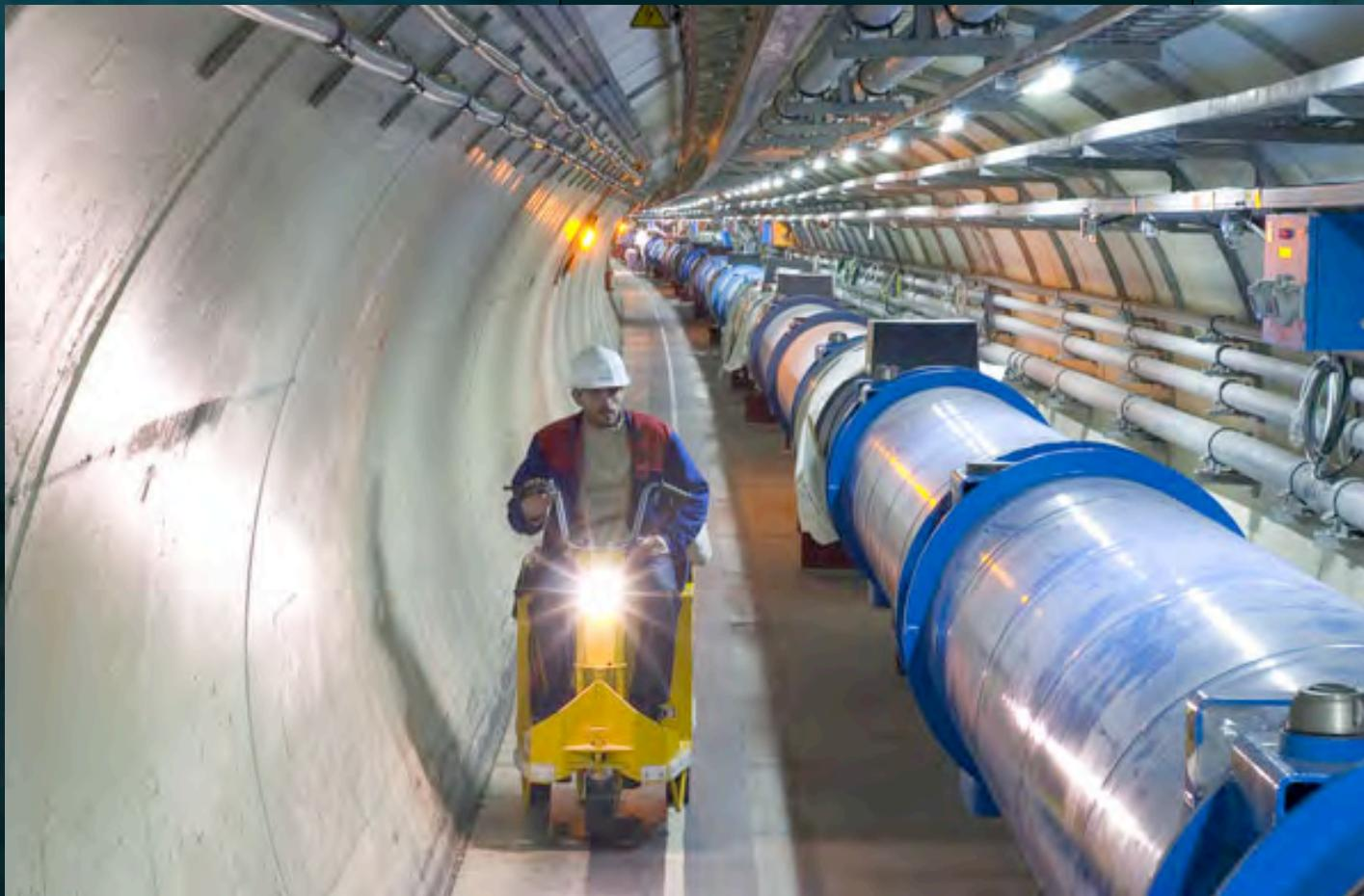
Several thousand billion protons traveling at 99.9999991% of the speed of light will travel round the 27km ring over 11000 times a second 100 m underground
